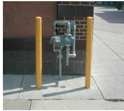
Bollards Installed to Protect
